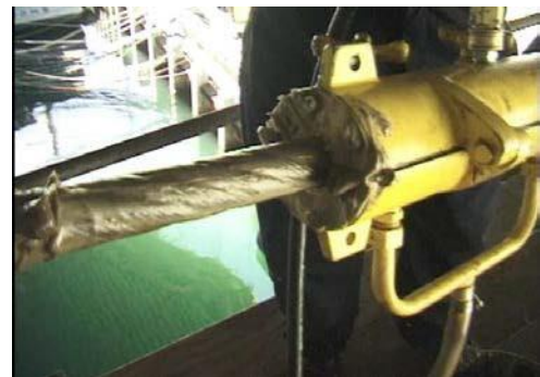
USS Stennis Aircraft Elevator Support Cables
