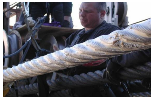
Hoover Dam – 76mm -Being coated with Dynagard E™
